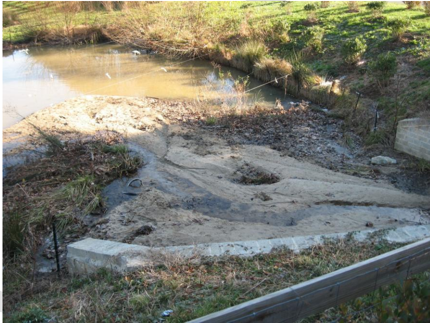
Figure 4.4 Sedimentation in Forebay
