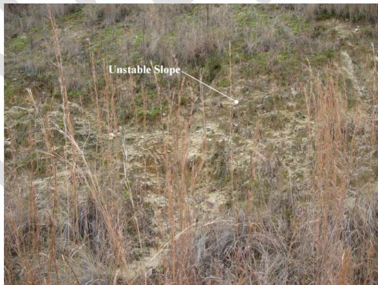
Figure 4.13 Slope Erosion
