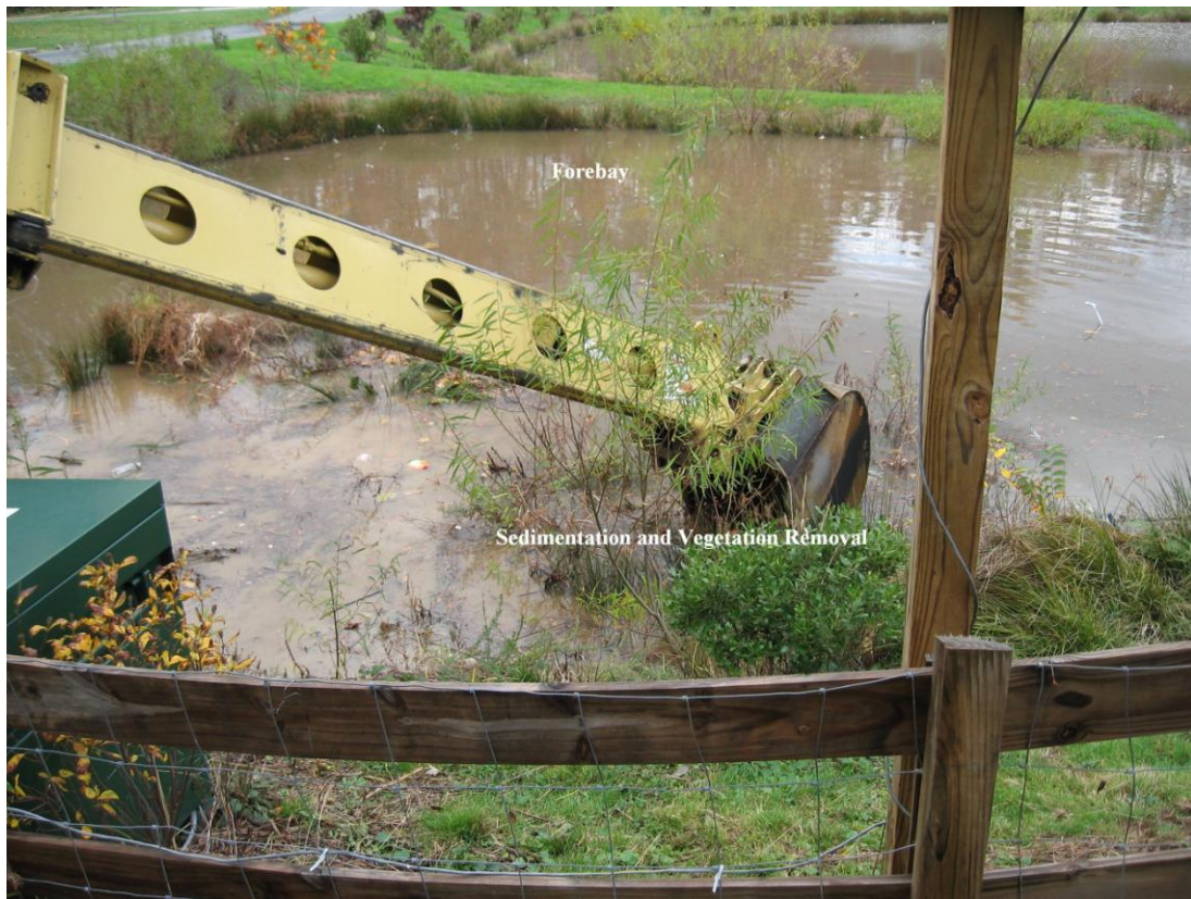
Figure 4.5 Excavating Forebay
