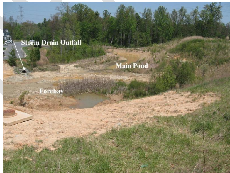
Figure 4.8 Wetpond Excavation
