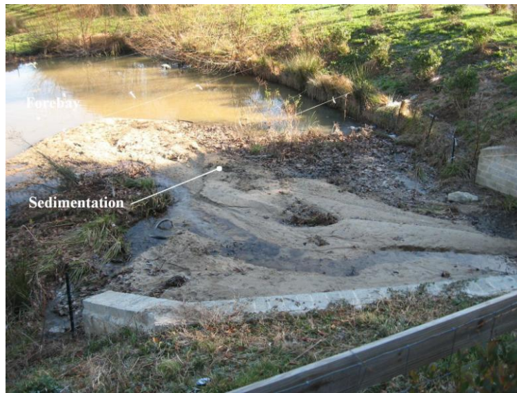
Figure 5.4 Sedimentation in Forebay
