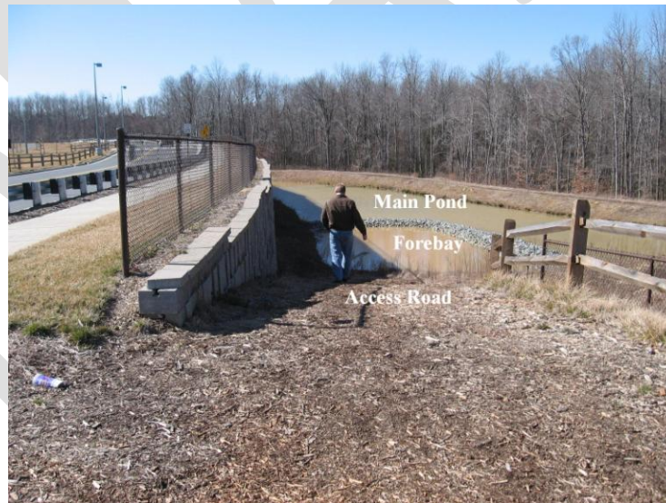
Figure 4.3 Maintenance Access Road
