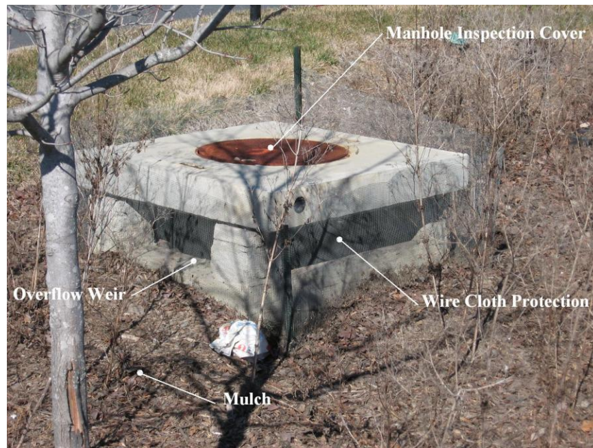
Figure 3.2 Overflow Weir
