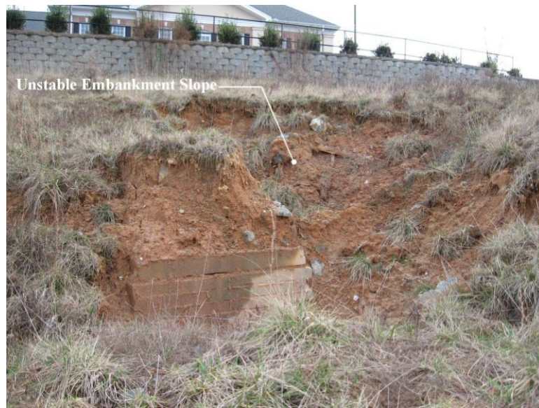
Figure 4.10 Embankment Erosion
