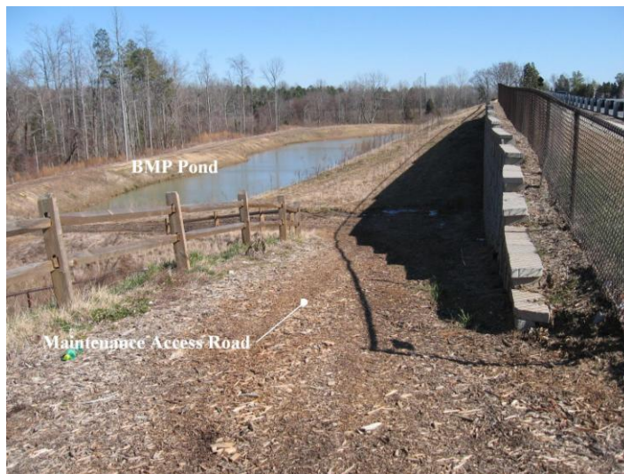
Figure 5.3 Maintenance Access Road
