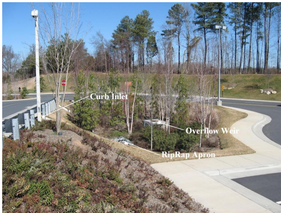
Figure 3.1 Well-maintained Bioretention Facility
