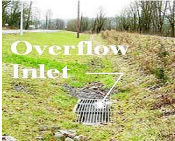
Figure 7.1 Filter Strip Inlet
