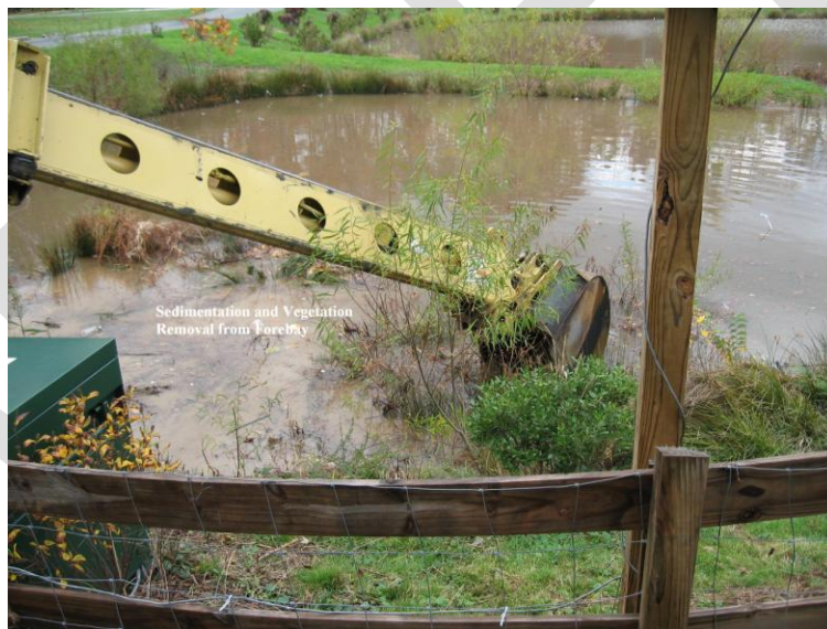
Figure 5.5 Excavating Forebay
