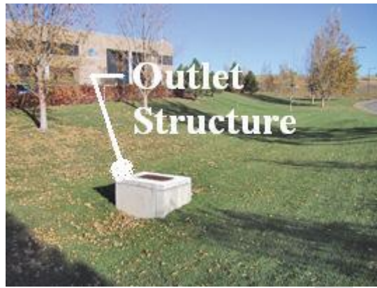
Figure 8.2 Well Maintained Detention Basin
